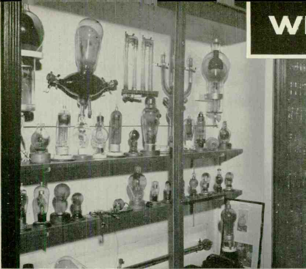
(Left) A collection of many early mercury rectifiers. In top row, partially hidden by cabinet upright, is a three-part rectifier patented by Steinmetz in 1915.
